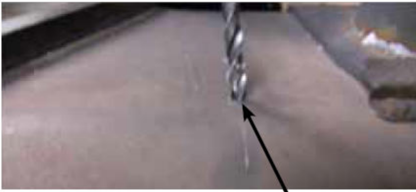
Drill hole with 1/4" drill bit
