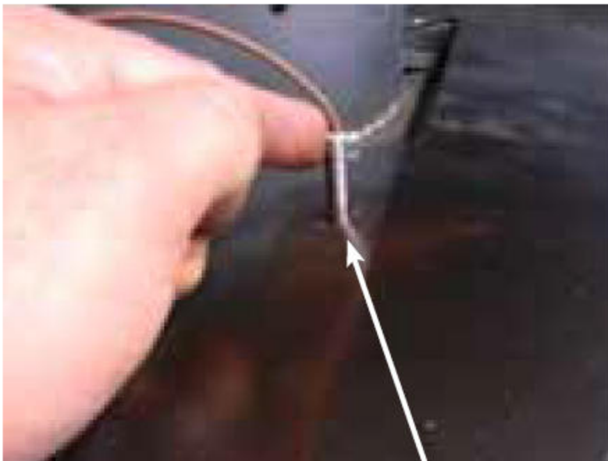
Install temperature probe
