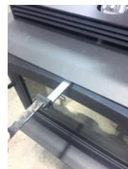
Bypass located above door
